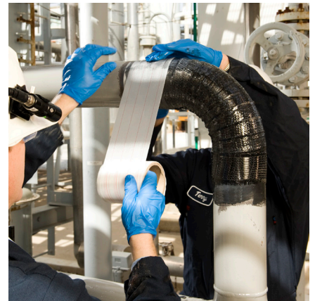
Prepare composite for topcoat.
