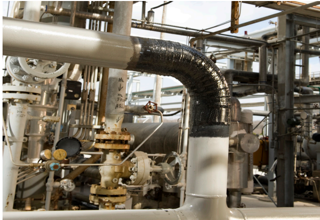
■ RES-Q® Composite Wrap for Process Piping Installation services and customer training available
